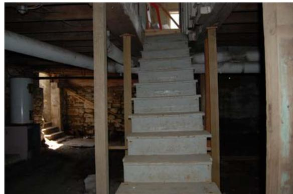
“opened up” when the basement was dug, or the staircase opening was created immediately upon the digging of the basement. There are 12 stairs making up the staircase supported by two stringers. The stringers are hung at the top end by nails only and land on crude stones. The stairs have round-nose treads and solid risers, but they are open on the sides lending to the concept that the stairs were not original construction and inserted later. There is no hand rail.
