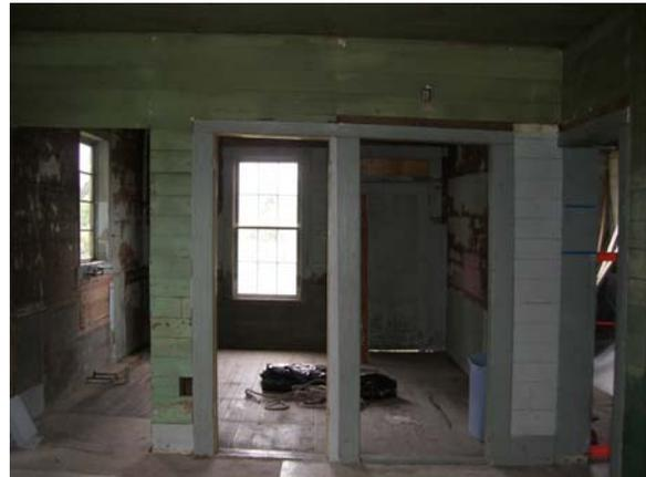
The center opening on the kitchen's west wall should also be filled-in again. This would require the removal of the casing on its left and top, again carefully documenting the materials that are removed. It would make sense to do this work in conjunction with the closure of the refrigerator hole. The small section of exiting tongue and groove between the openings could then be removed and both holed filled at the same time, restoring a continuous wall surface.
