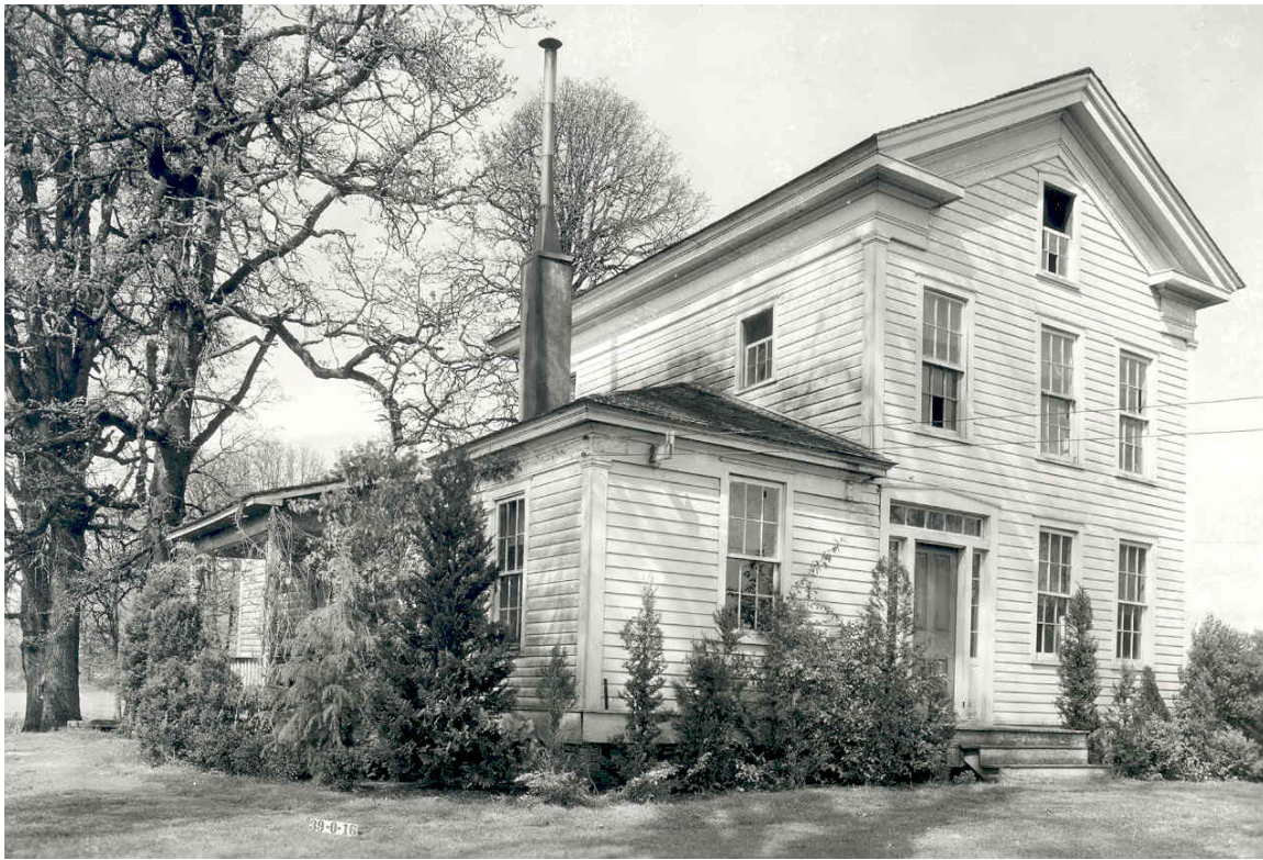
Figure 7. This one of two 1934 Historic American Building Survey (HABS) photos taken of the house. An open south porch has been constructed to shelter the entry. This is the best photo of the tall chimney flue serving the kitchen (and possibly the living room) and of the southeast 6/6 windows before removal.
