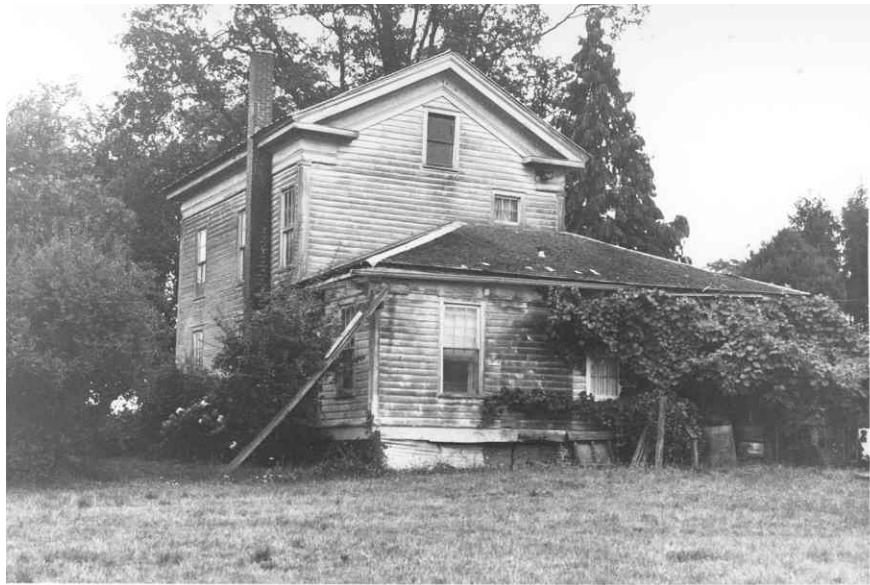
Figure 10. This is the rear of the house in 1971. The gable structure used to protect the basement stairs has been removed, along with its stairs and opening, but its shadow remains. Both the west and north exterior doors are completely overgrown.
