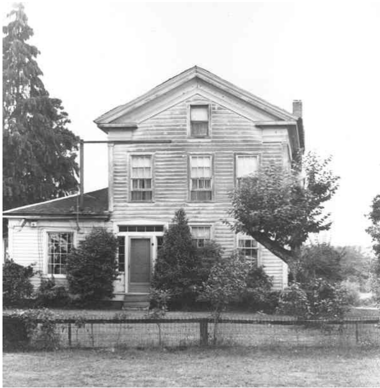
Figure 9. This is the front of the house in 1971. The kitchen/living room chimney flue has been removed and the window to the left of the front door substituted for a larger 16-pane fixed window.
