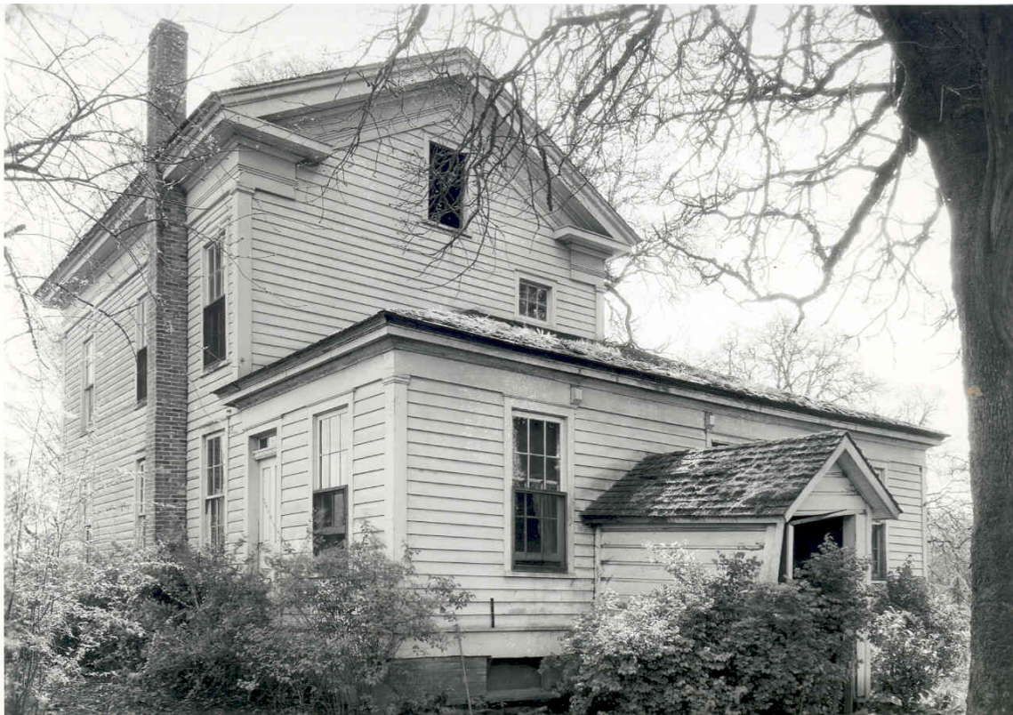
Figure 8. This is the second of two 1934 HABS photos taken of the A.T. Smith House. This shows the rear of the house along with the exterior chimney that replaced the original interior chimney and was installed to vent the basement furnace in the late 1920s. Also visible is a collapsing gabled structure used to shelter the basement entrance.
