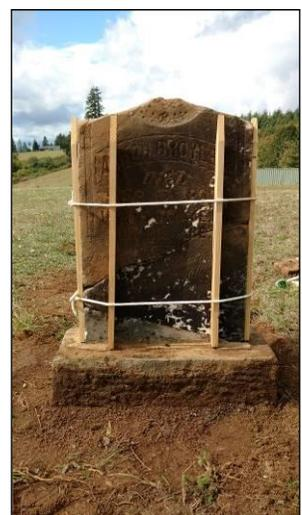
repair can be touched within 30 minutes; however, ideally braces should remain in place for a full seven days while the epoxy cures.
