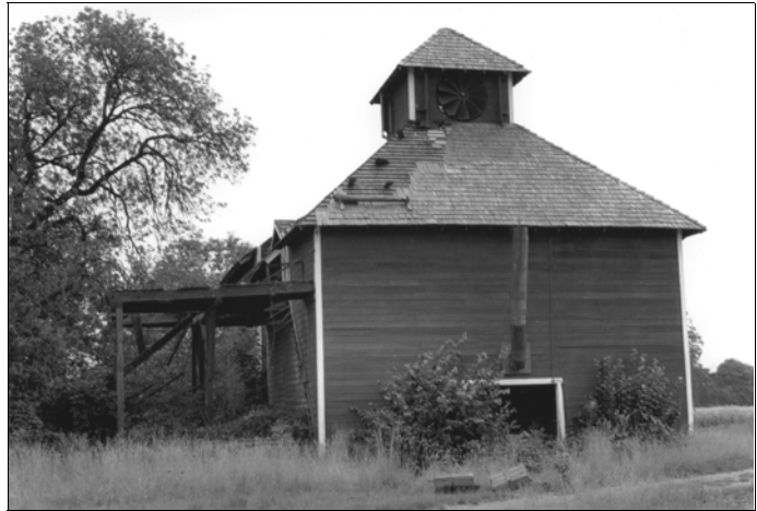
Hop barn in the River Road area. Demolished. Photo courtesy of Lane County Historical Museum (GN2053)
