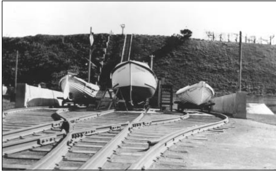
Figure 95. Remains of the Coquille River Life-Saving Station Boathouse After Bandon Fire, 1938. Source: U.S. Coast Guard Headquarters (Coquille River File).
