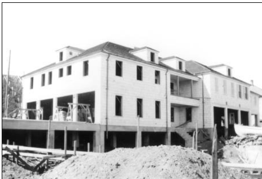
Figure 96. Coquille River Lifeboat Station Under Construction, 1939. Source: U.S. Coast Guard Headquarters (Coquille River File).
