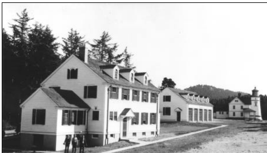
Figure 110. Umpqua River Lifeboat Station, 1939. Source: U.S. Coast Guard Headquarters (Umpqua River File).
