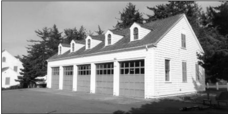
Figure 113. Equipment Building at Umpqua River Lifeboat Station, 1991. Source: Oregon State Historic Preservation Office (Umpqua River Coast Guard Station File).
