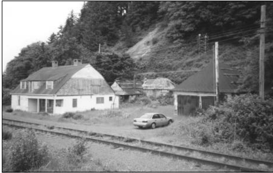
Figure 159. Tillamook Bay Life-Saving Station (1907) in 1997. Source: Author.
