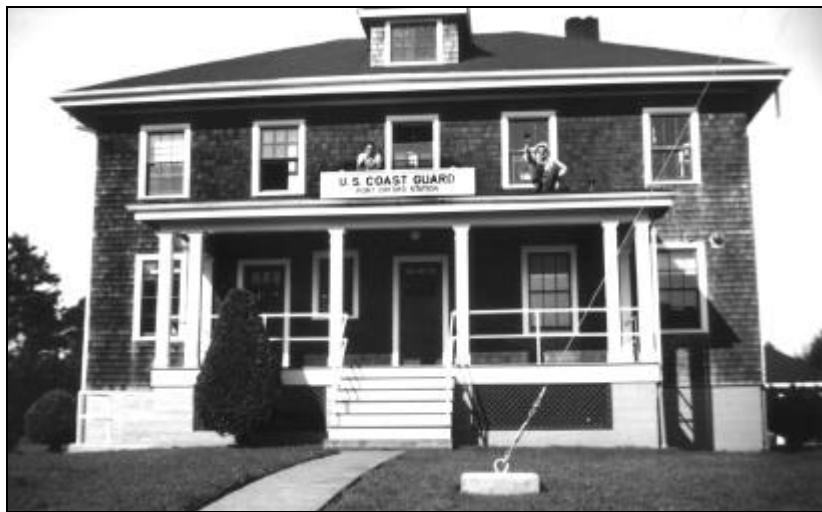
Figure 174. Station House, Port Orford Lifeboat Station, Circa 1940. Source: Oregon State Historic Preservation Office (Port Orford File).
