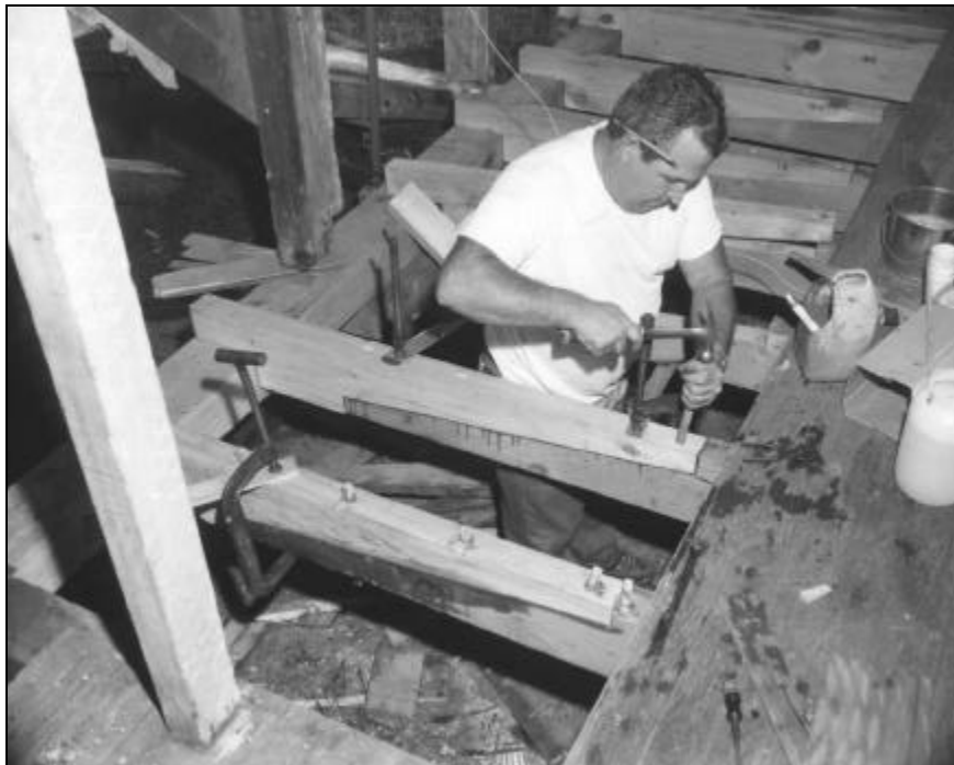
Figure 184. Splicing Floor Joists at Block Island Life-Saving Station, Rhode Island, 1970. Source: Mystic Seaport (#70-8-364).
