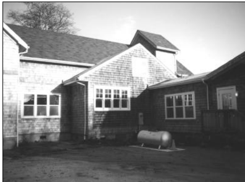
Figure 192. Keeper's Dwelling (1915) Enveloped, Coos Bay Lifeboat Station, 1999. Source: Author.
