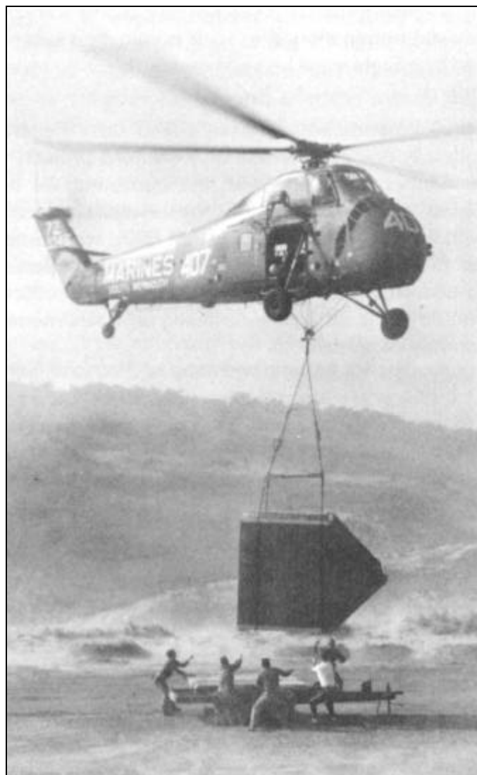
Figure 188. Marine Helicopter Moving Halfway House at Mystic Seaport in 1968. Source: Curtis, Moving Historic Buildings .
