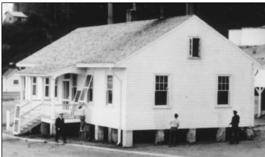
Figure 182. Removing Screens and Washing Windows, Coos Bay Lifeboat Station, 1923. Source: U.S. Coast Guard Headquarters (Coos Bay File).
