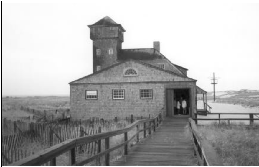
Figure 190. Old Harbor Life-Saving Station (1898) in New Context at Race Point, Massachusetts, 1997. Source: Author.
